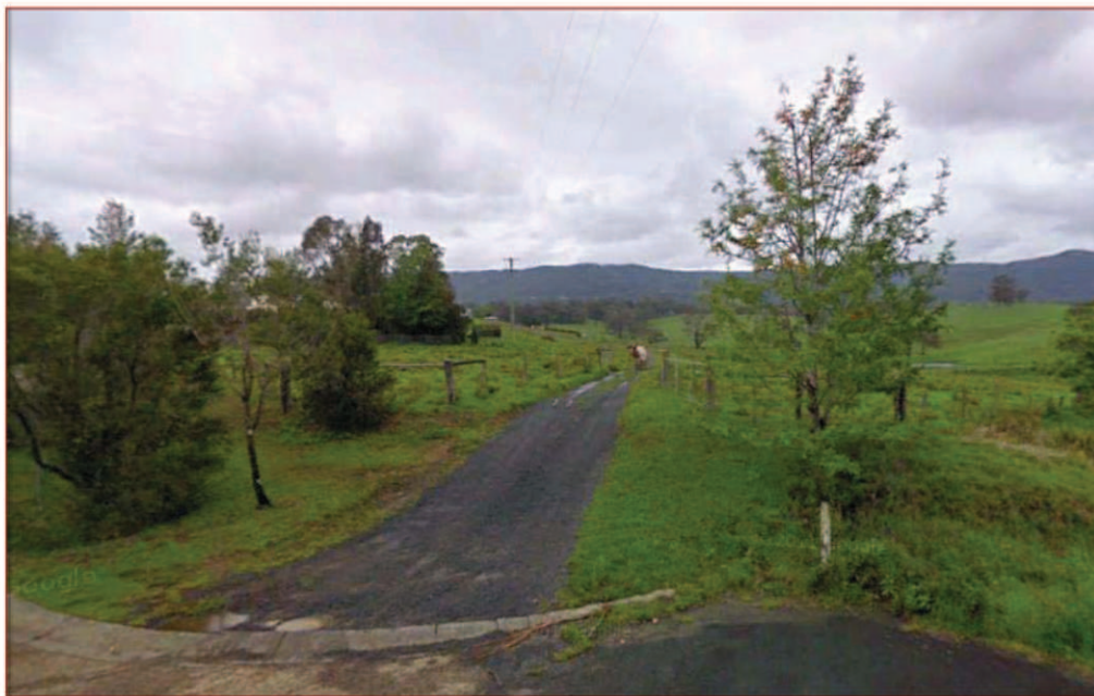
Figure 13: View south from Dualla Road/Downes Place intersection.
